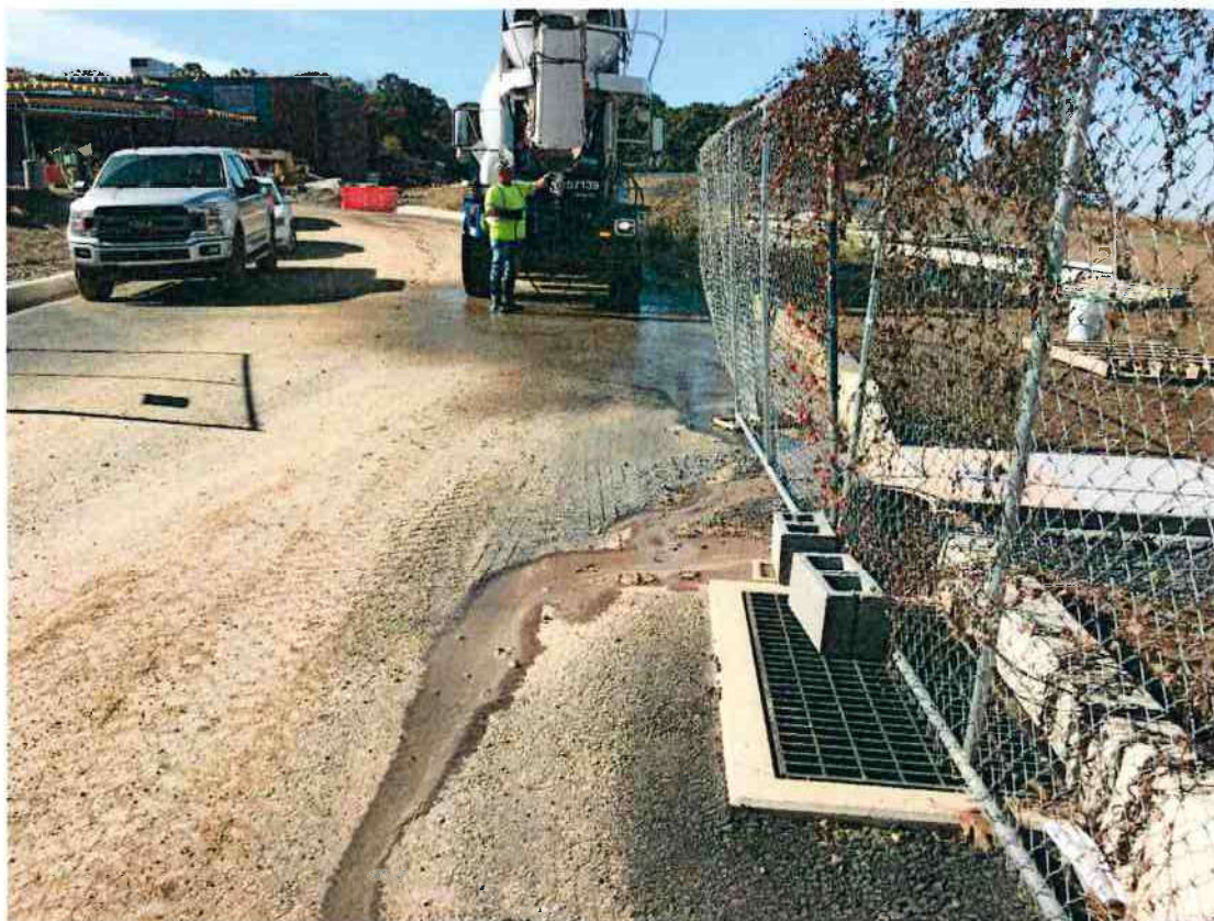
Photo #2 – Pennsy Supply Truck being washed in the street and discharge entering the storm inlet.
